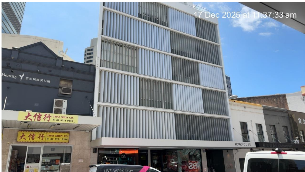
Figure 1: 398-402 Sussex Street, Haymarket, viewed from the south-west
